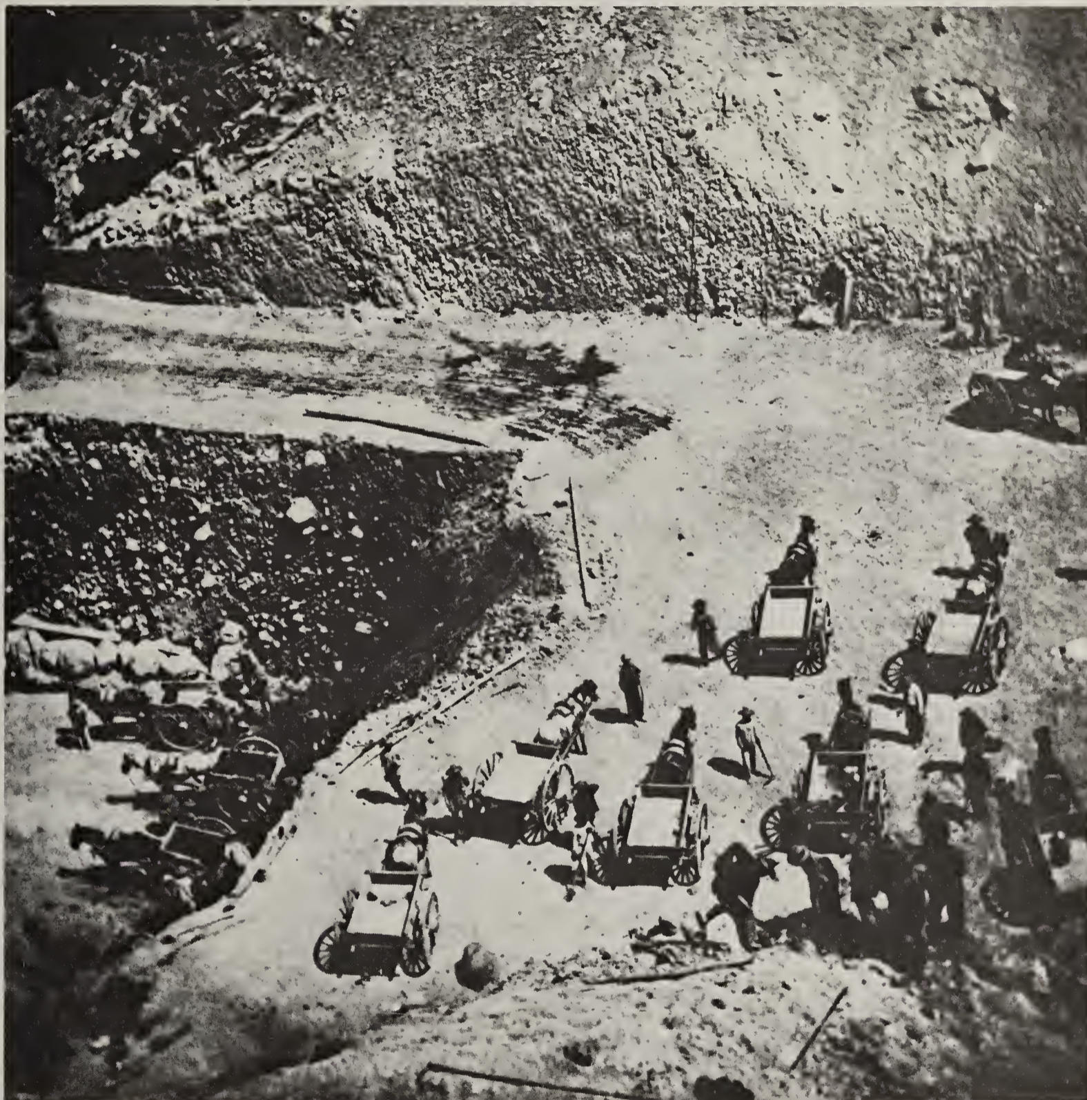
Figure 8: Chinese work gangs, horse-drawn carts, and hand tools accomplished much of the grading work (Southern Pacific, Alfred A. Hart Photograph).
